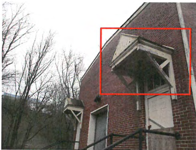
The Wooden Soffit and Fascia Components were found to utilize Lead-Based Paint
