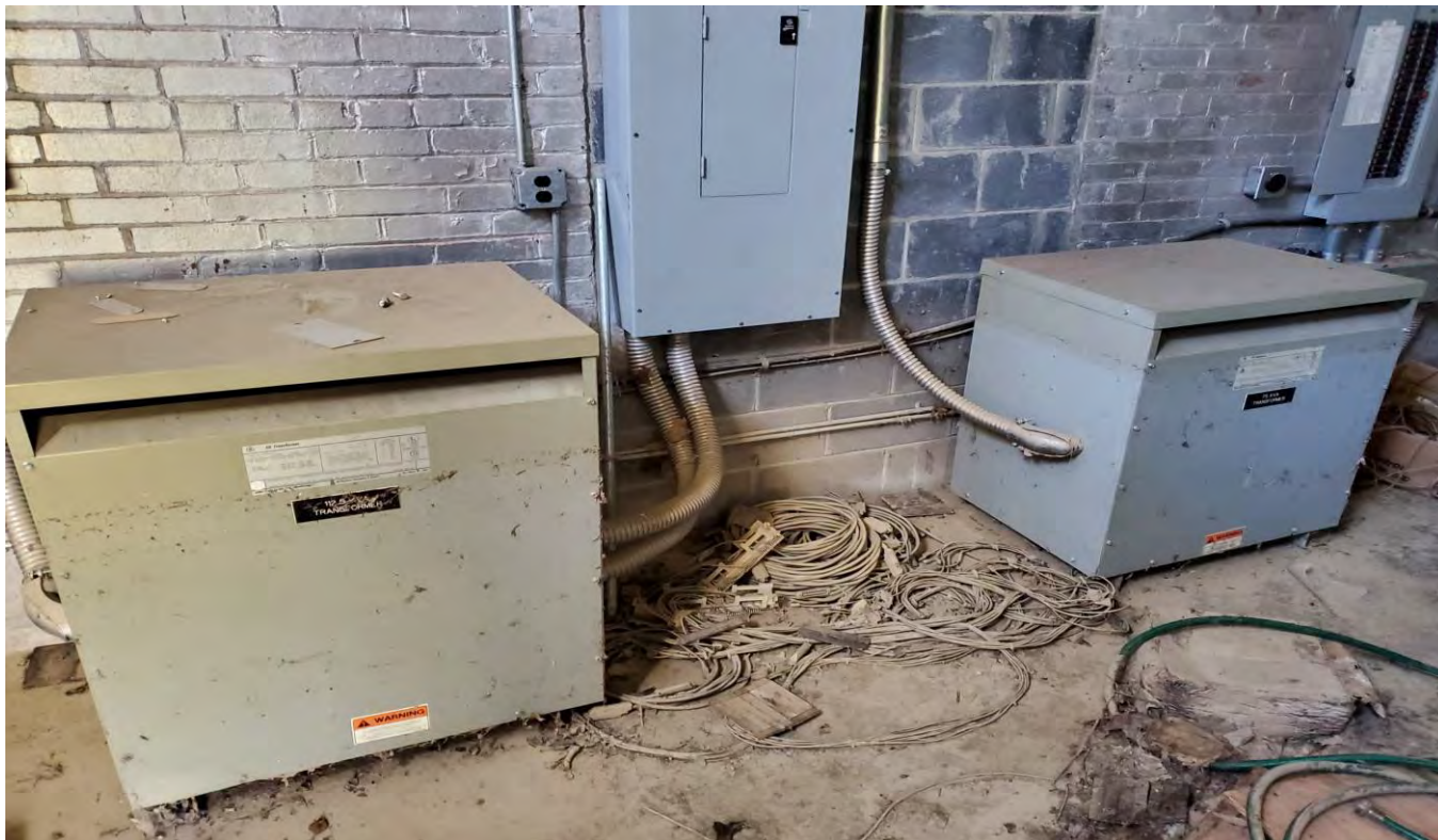
PHOTOGRAPH 13. Two transformers in the former boiler room / now electrical room, Calfee School Building.
