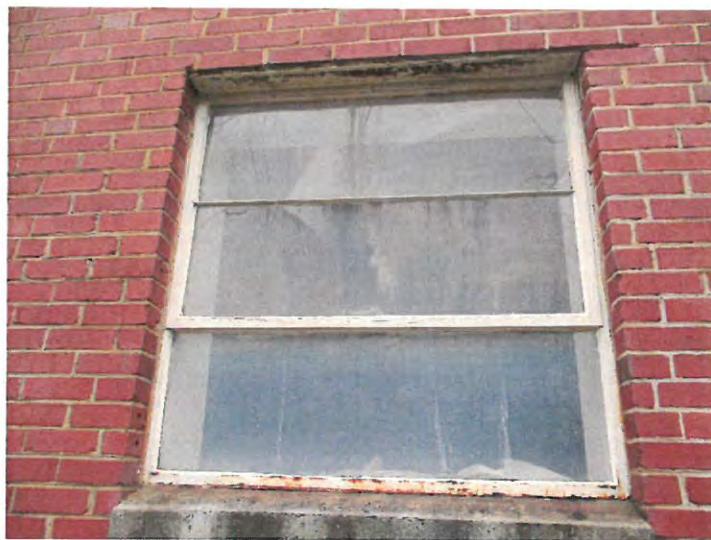
The metal-framed windows were found to utilize Lead-Based Paint
